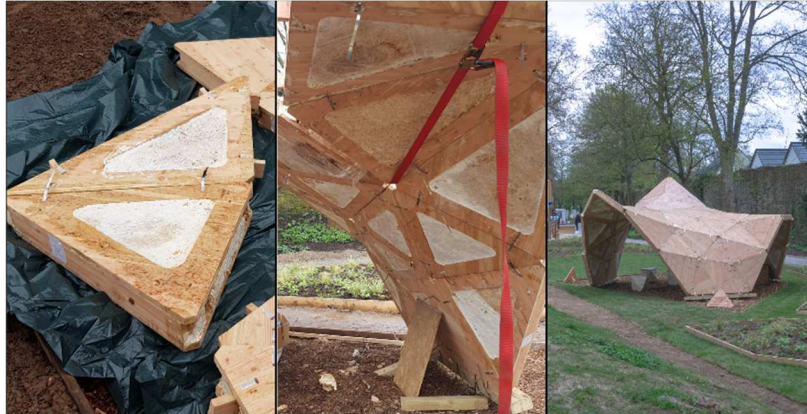
Figure 7. Phase 02 - From left to right: Two triangular elements already joined with the cross spacers and stainless-steel strap; Construction of the pavilion; and Final assembly of the pavilion. Source: Author, 2023.
